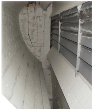
Ceramic liners after 7 years of usage
